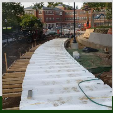
Geo-Joist helps reduce the amount of concrete needed to span large distances like this elevated walkway at U of R University, while increasing the strength of the slab due to its innovative engineering.
