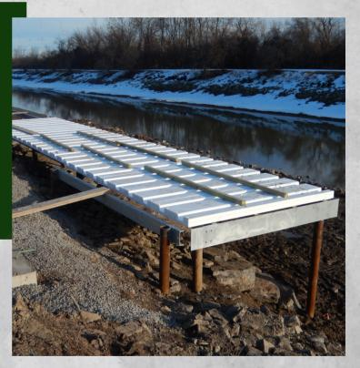
Above: A Geo-Joist dock along the Erie Canal, NY. Geo-Joist was a perfect solution for this dock, because of its ability to span large areas without excessive weight from extra concrete.
